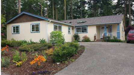
Renovations are complete!
